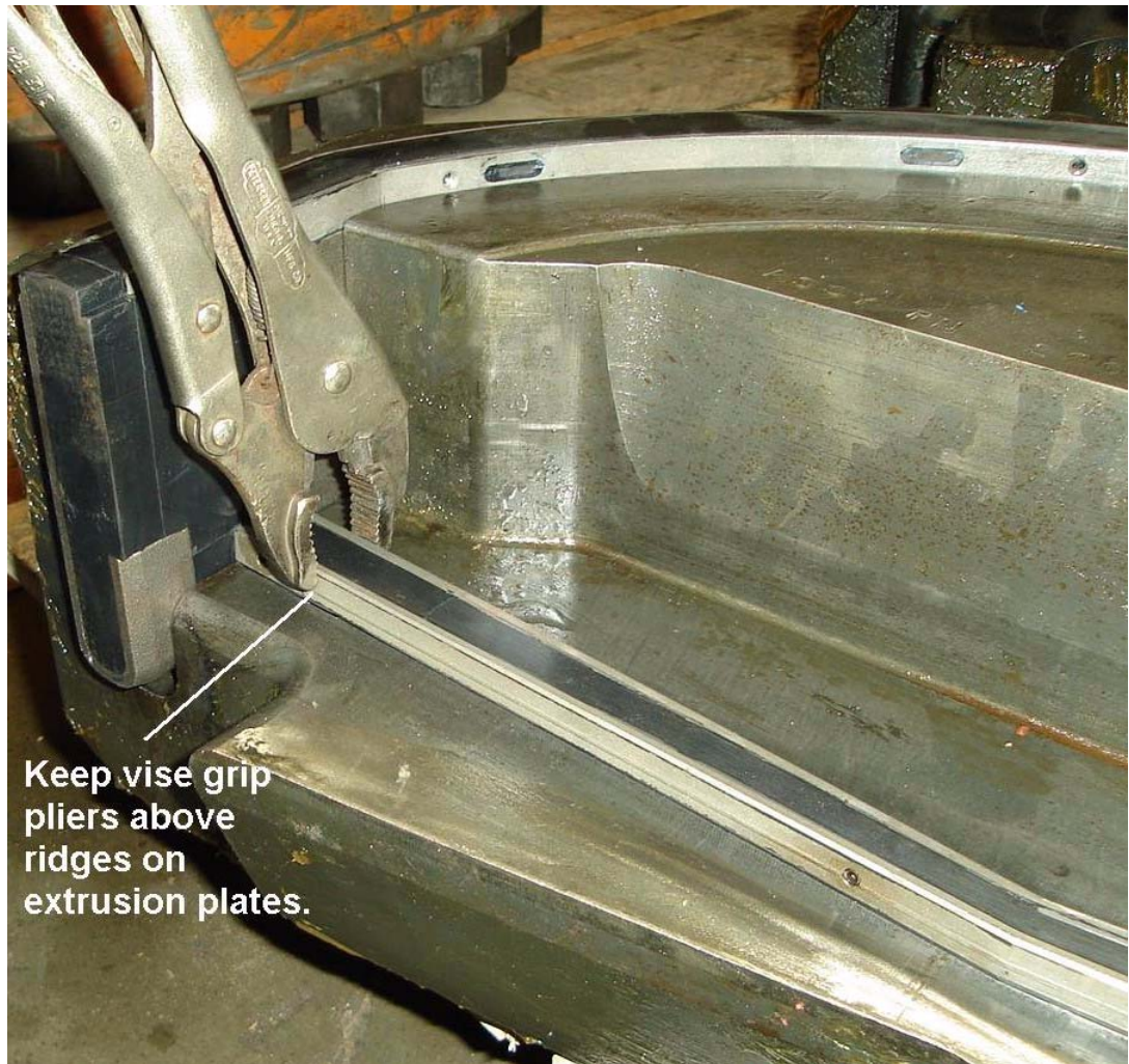
Figure 5-86. Compressing Extrusion Plate
