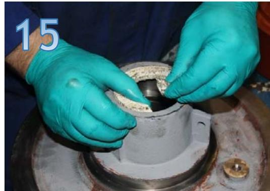
**15.** Install rope packing (Picture 15) in stuffing box.
